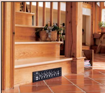
Twin-Flo III heater staircase installation.
