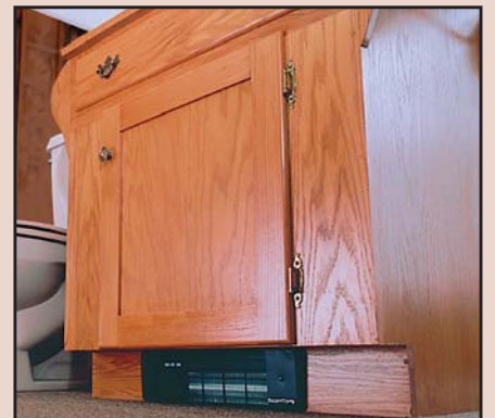
Twin-Flo III heater bathroom cabinet installation.
